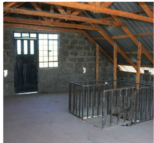
Above: Attic room to balcony, before sub-division
